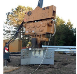
Hanging Vibratory Hammer - Excavator
