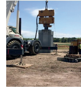
Hanging Vibratory Hammer - Crane
