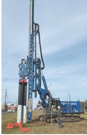
Louisiana Department of Transportation Federally funded project Installed Eight (8) Friction Piles over eight (8) miles for Monopoles standing 65' - 110' tall
