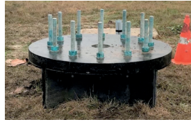
Louisiana Department of Transportation Federally funded project Installed Eight (8) Friction Piles over eight (8) miles for Monopoles standing 65' - 110' tall
